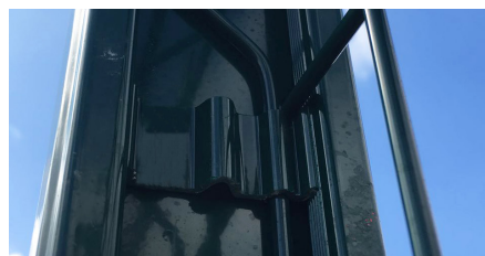
CLIP FIXATION POTEAU/PANNEAU
